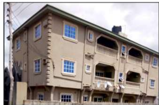
Plate 1: Typical view naturally ventilated building in the study Area Source: Field work (2022).
