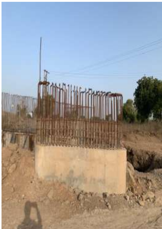
Figure 1.1: Partially completed column structure of NH-6
