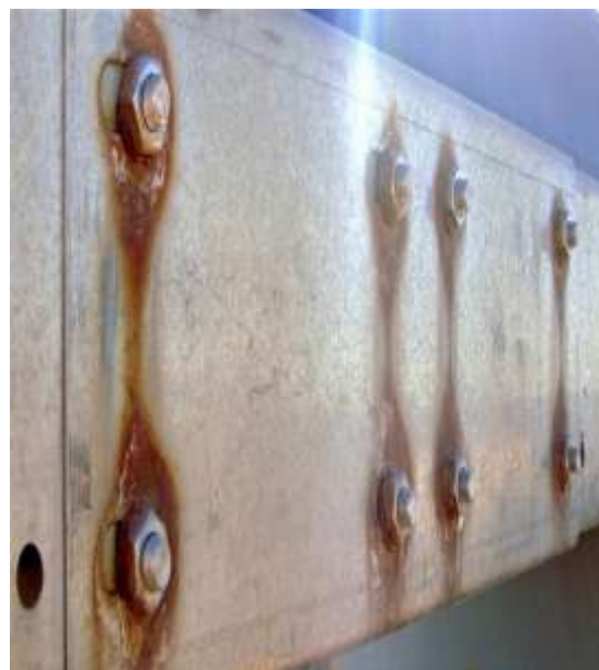
Figure 1.3: Galvanic corrosion
