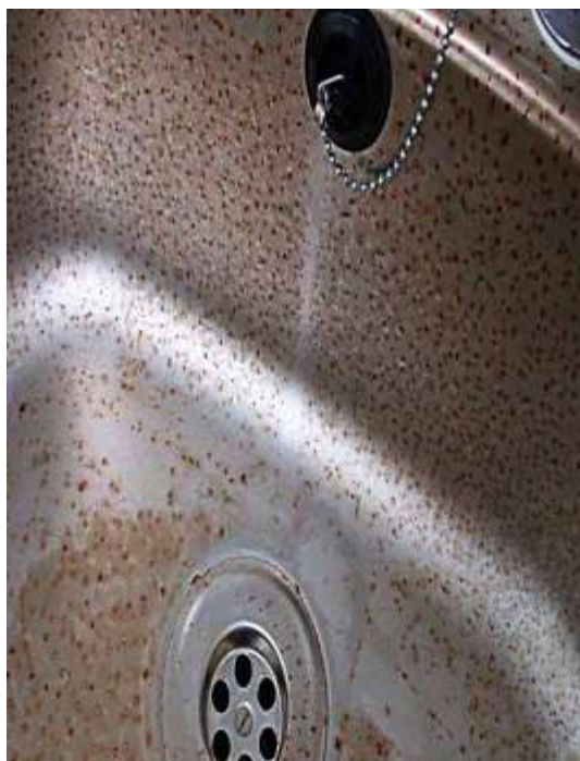
Figure 1.6: Pitting corrosion on sink surface
