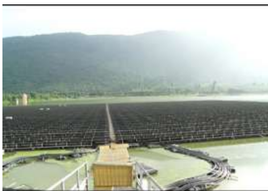
FLOATING SOLAR POWER PLANT
