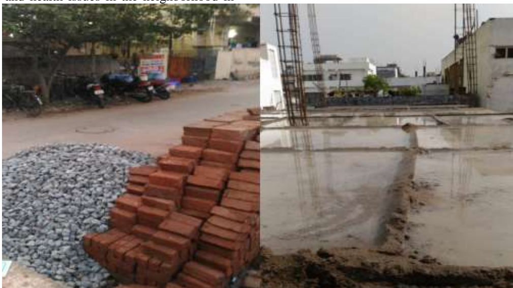
Figure 8: Stacking bricks and stone on street (left), Curing ponds are favorite spots for mosquito breeding (right)
