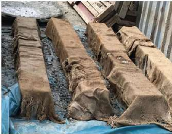
(Fig No. 3 curing of concrete beam)
