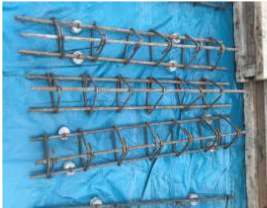
(Fig No. 2 triangular shape stirrups reinforcement)
