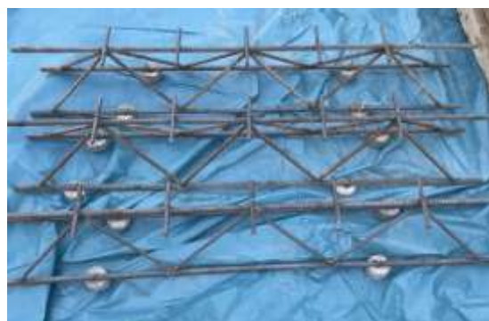
(Fig No. 2 Lattice reinforcement)
