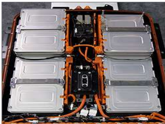
Fig. 5. Battery compartment of Present electric car. Showing smaller batteries connected together to make single battery
