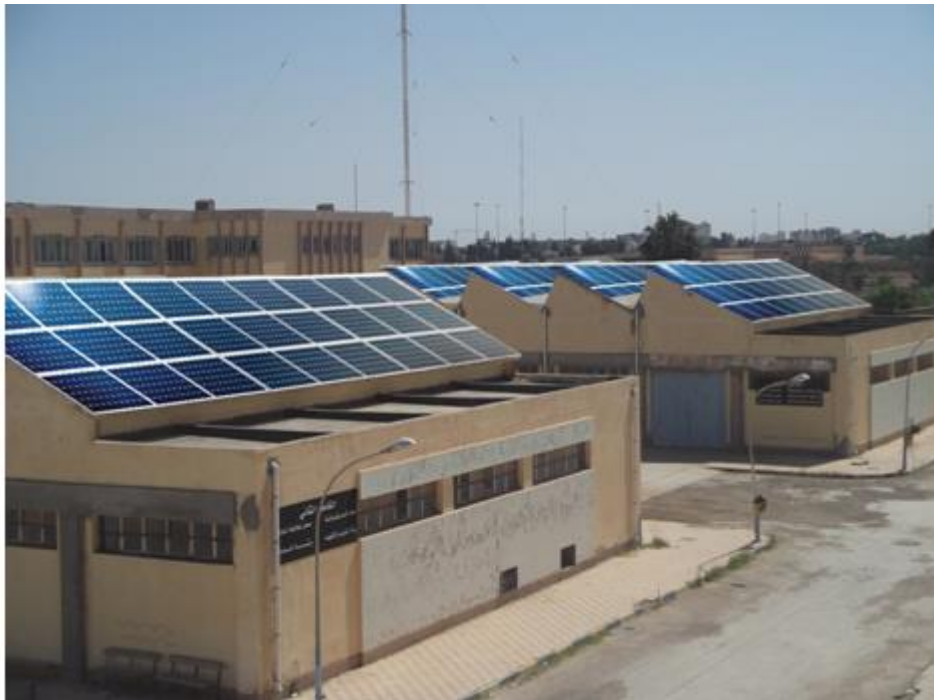
Figure (8) The default format for the installation of matrimonial plates on buildings.
