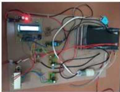
Fig. 4 Fast Charging of Battery by using copper tube cooling system.
