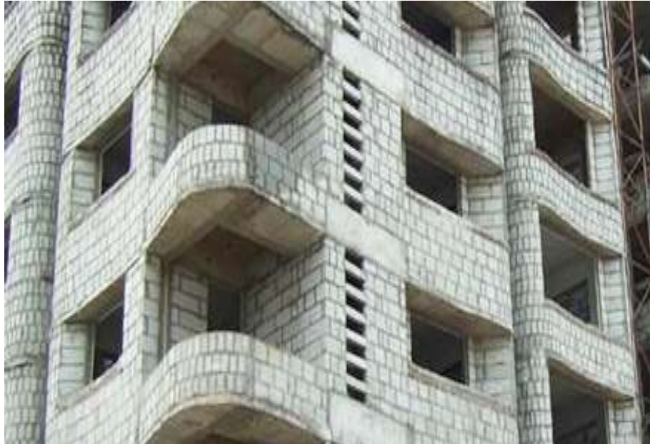
Fig .1.2 Building constructed with AAC blocks
