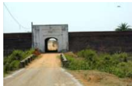
Fig 2 : Entrance gate of the fort
