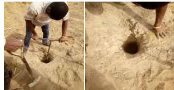
Plate I: Boring Using Hand Auger Plate II: Bored hole
