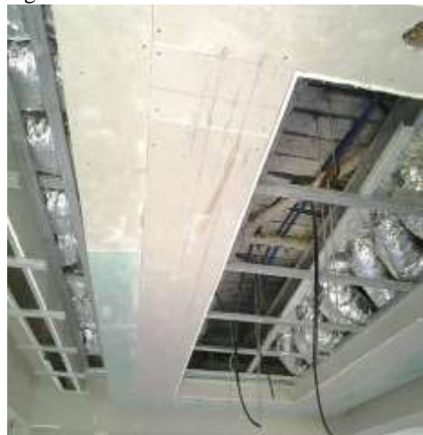
Fig 8. CONCEALED MECHANICAL AND ELECTRICAL INSULATION
