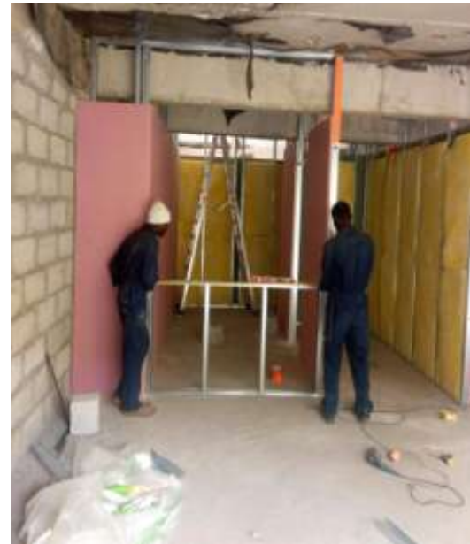
Fig 2 DRYWALL INSTALLATION IN PROGRESS
