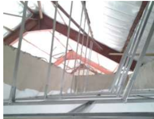
Fig 4. INSTALLATION BY PROFILE METHOD
