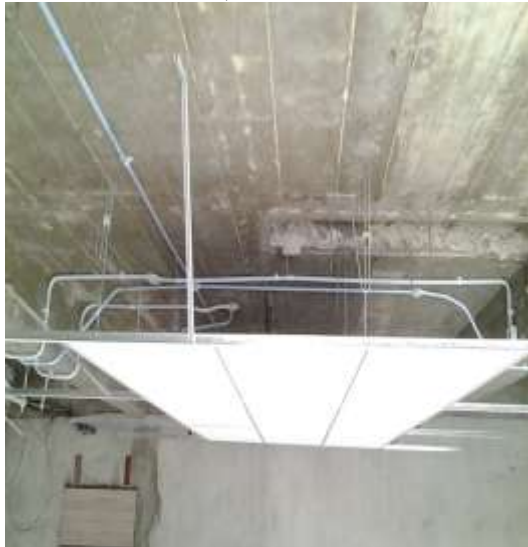
Fig 3. Sample of Installation by Grid Method
