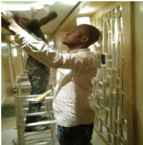
Fig 7. ACCESS PANEL INSTALLATION
