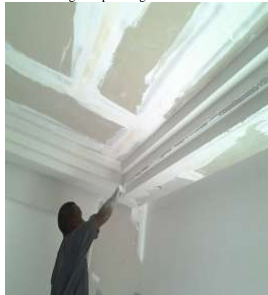
Fig 9: SKIMMING WORK IN PROGRESS
