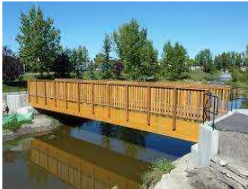
Glulam pedestrian bridge
