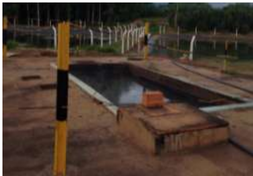
Fig. 2.1 – Liquid effluent treatment installation
