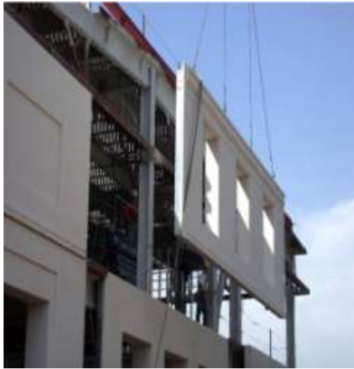
Figure 1.1: Construction stage of a precast wall panelled building
