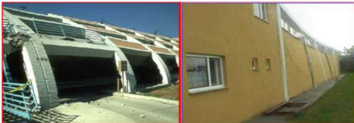
Figure 3. Failure of irregular structures
