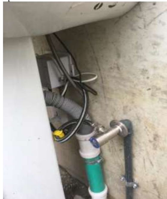
Plate 2: Pictorial diagram of the water inlet and the sensor signal wire.
