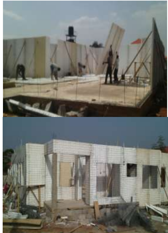
Figure 3.2: Handling and Installation of EPS panels
