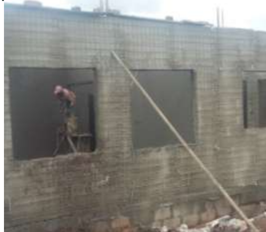
Figure 3.1: Shotcreting of EPS panels
