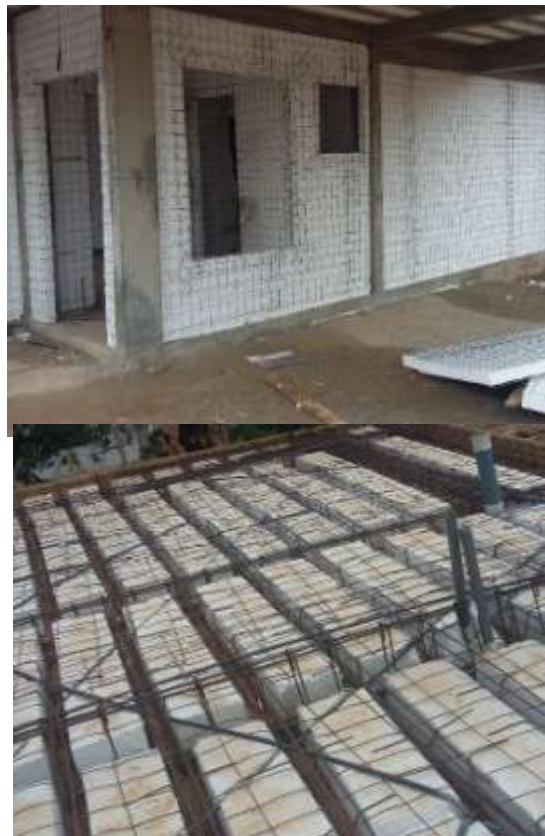
Figure 2.1: Wall and Slab constructed of EPS panels
