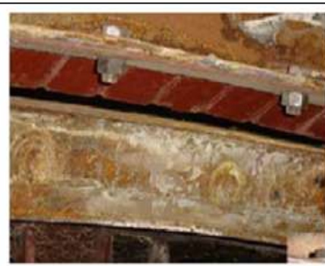
Figure 3. Thin sealing plates for improvement of circumferential sealing
