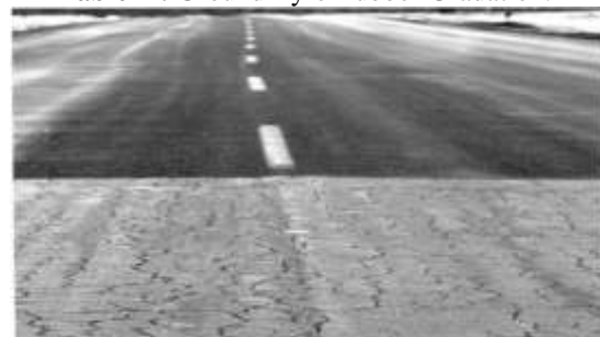
Fig: Rubberised bitumen chip seal applied to badly cracked pavement.
