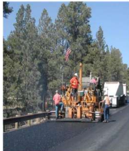
Fig -6: Rubberised bitumen construction.
