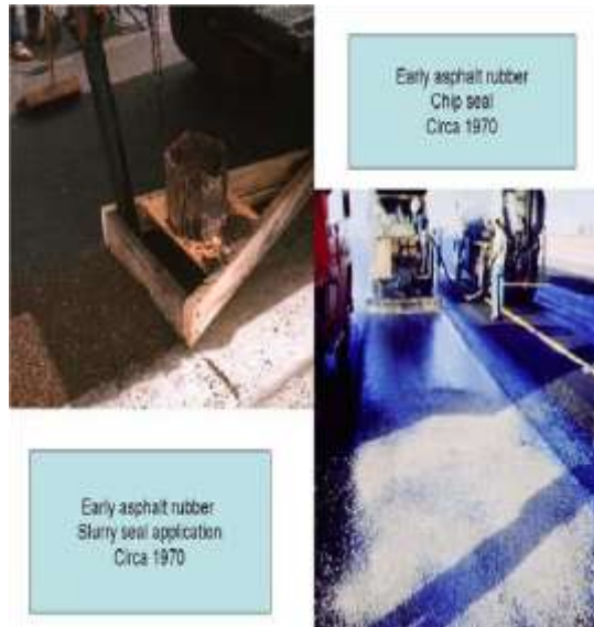
Fig -1: Rubberised bitumen applied as a slurry seal
