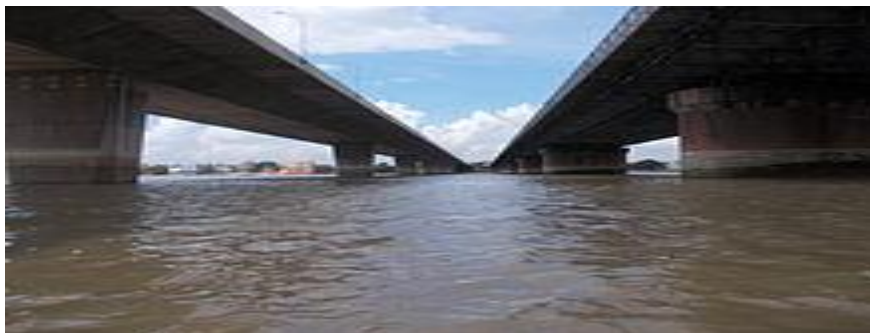
Twin bridges: 2007 Nivedita Setu (left) and 1932 Vivekananda Setu (right), from the Hooghly River
