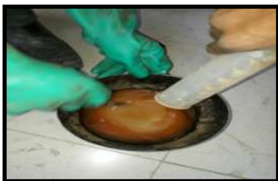
Fig. 3 Preparation of Primer by Mixing Primer and Hardener
