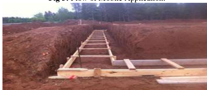
Fig 4: The image of Site progress photo uploaded by site engineer.
