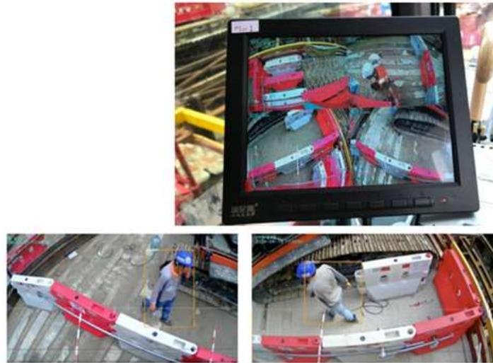
Fig 1: Safety monitoring of heavy machinery operations
