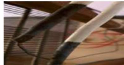
Figure : 2.3.3 Capillary Tube
