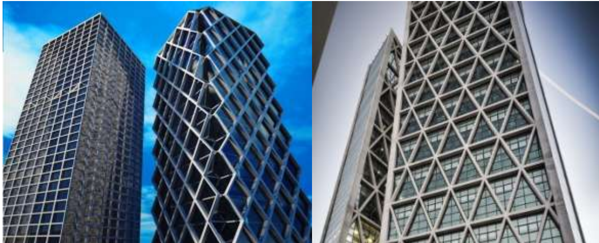
Fig 1 – Diagrid Structural Building
