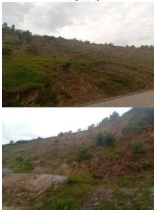
Landslide in Bushhoki Sector
