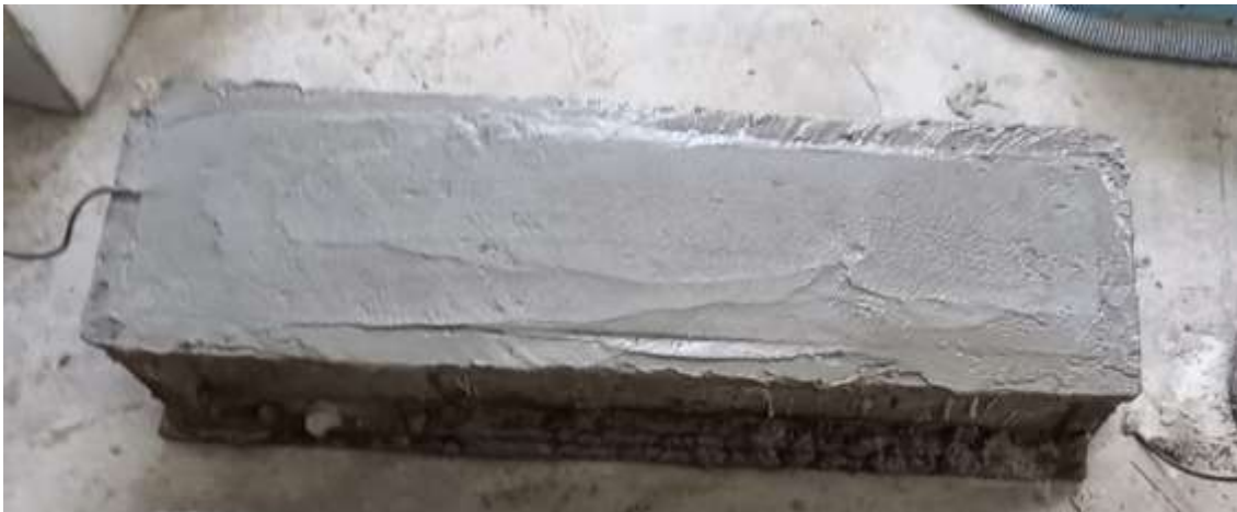
Figure 2 : View of beam at the time of casting process
