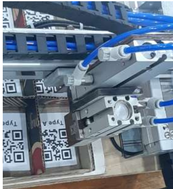
Figure 3.3. PLC controls the AC Servo and pneumatic systems to place products in their respective positions
