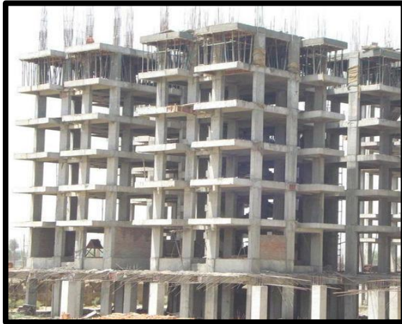
Figure 11: Typical example of RCC Framed Structures
