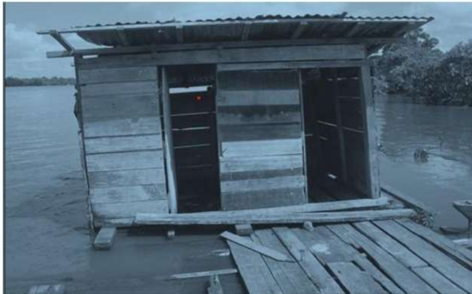
Figure 1: Exterior of hanging pit latrine
