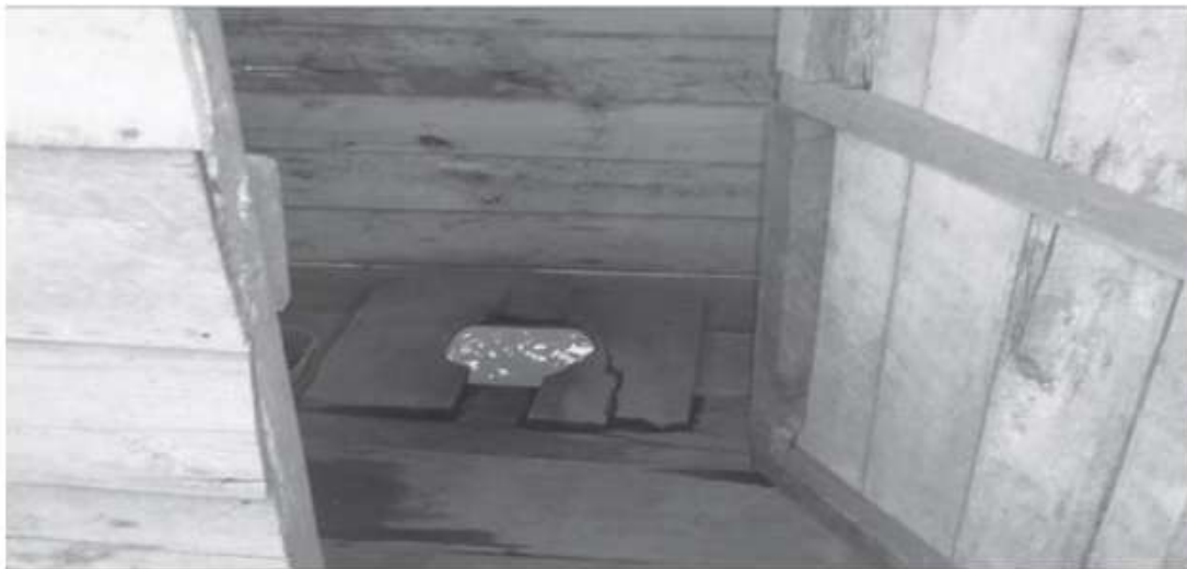
Figure 2: Interior view of hanging pit latrine
