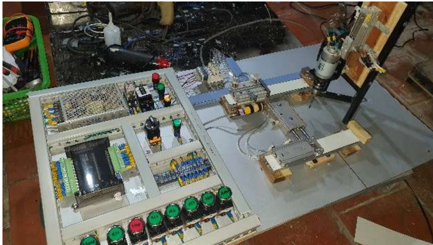
Figure 12. The image of the system after complete
