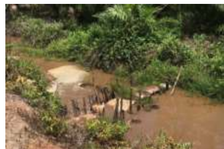
Figure 1. Condition of oil palm footbridge
