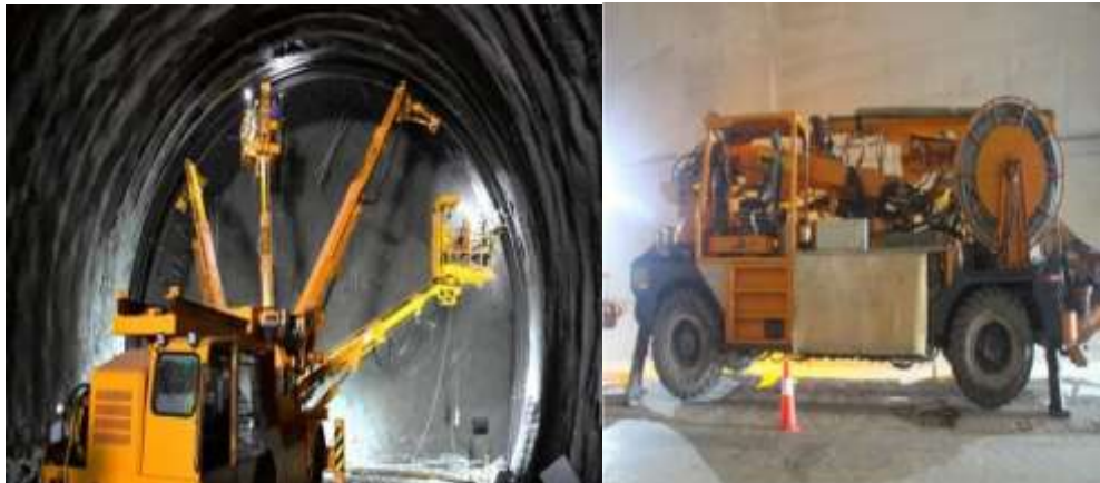
(a) Arch installation machine (b) Wet spraying machine
