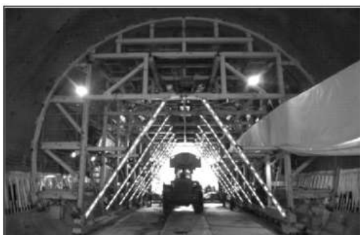
Fig. 3 Waterproof Board Laying and Hanging Trolley
