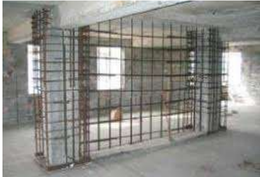
Fig 1.2 Adding Shear wall
