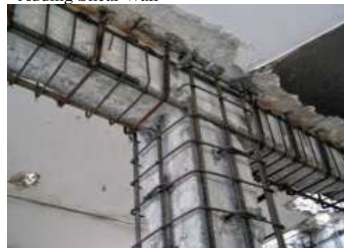
Fig 1.1 Jacketing of beam and column
