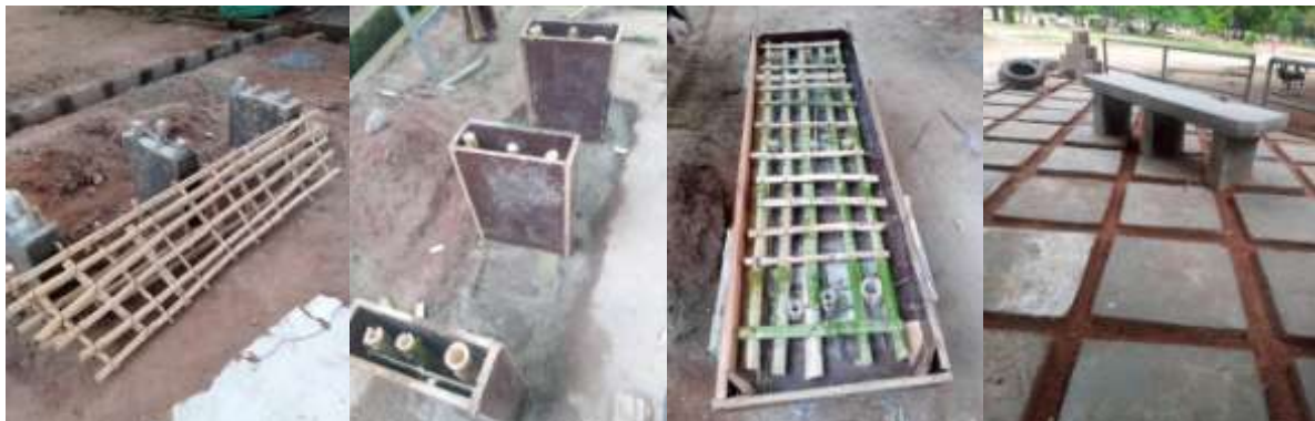
Step in construction of bamboo reinforced concrete bench Fig1,2,3 and 4
