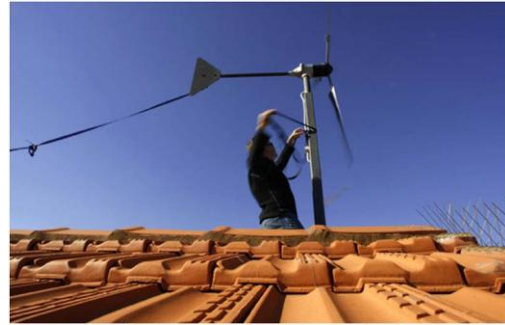
Figure 2. Installation of a wind turbine combined with a heat suction bridge
