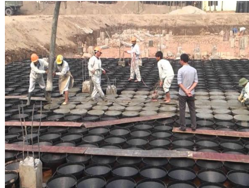
CONCRETE PLACEMENT USING PUMPS AT THE PLASTIC FUNNEL MOLD LOCATIONS
