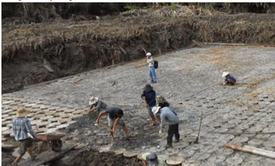
FILLING AND COMPACTING CRUSHED STONE TO CREATE THE TOP-BASE STRUCTURE
