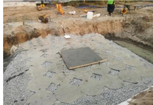
STRUCTURE OF THE TOP-BASE FOUNDATION [1]
