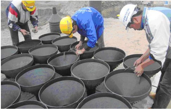
INSTALLATION OF PRECAST PLASTIC FUNNEL MOLDS
