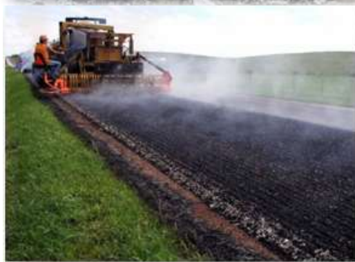
Figure 1 Hot In-Place Recycling
