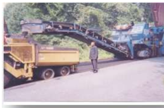
Figure.2. Cold In- Place Recycling (CIP)
