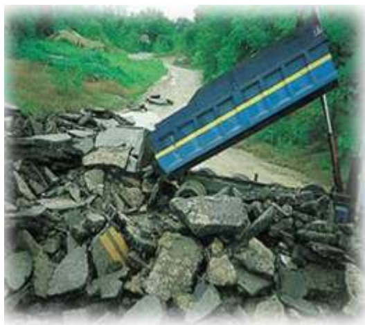
Figure.3. Central Plant Recycling.
