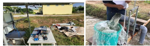
Figure 9: Pumping system and flow measurement and sampling equipment.
