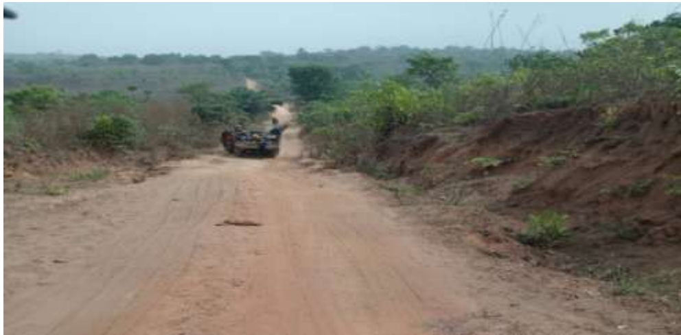
PLATE 1: Condition of road between Ifon and Aboluwodi camp.
