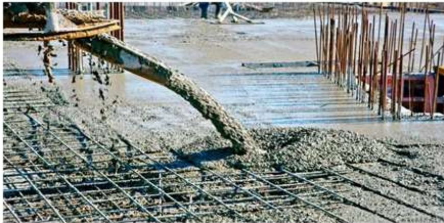
Fig 1: Self Compacting Concrete (SCC)
