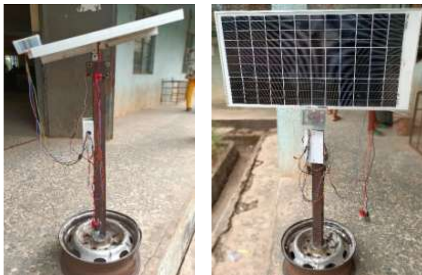
Figure 4 The complete assembly of the dual axis tracking device
