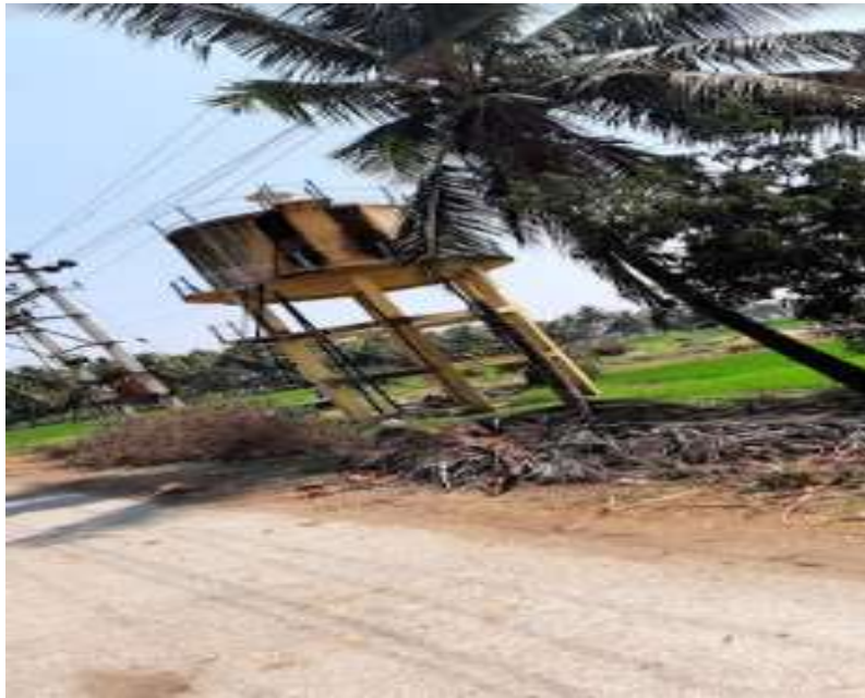
(fig,1.3: OHT for storing treated water).
