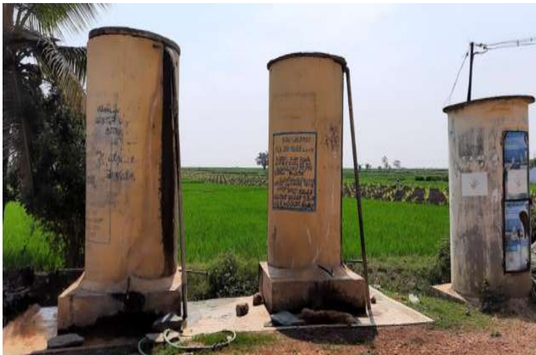
(fig,1.2: GLSR Tanks)
