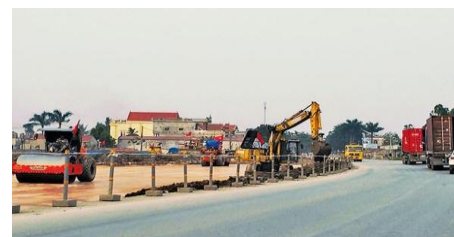
Renovate and upgrade National Highway 10
