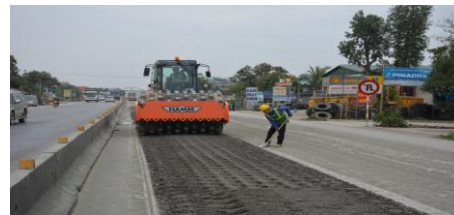
Treating wheel ruts
