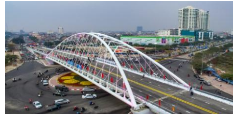
BigC – Le Hong Phong overpass
