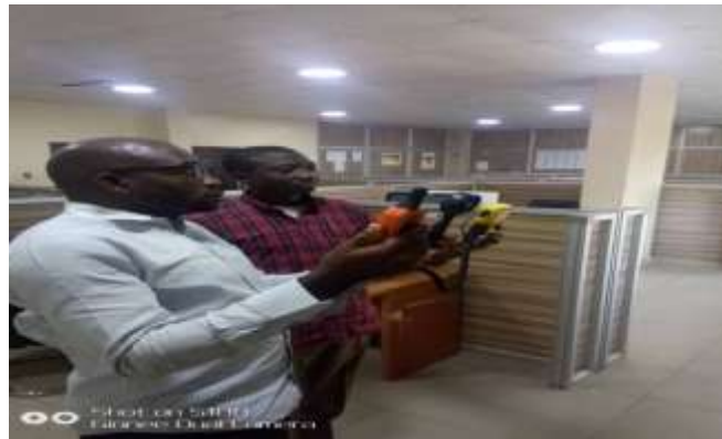
Figure 11: Team Members Taking Thermal Comfort Reading Using Anemometer, Humidity, Moisture and Temperature Sensors.
