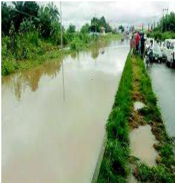
Figure 5: Flooding on Iworoko Highway 2018
