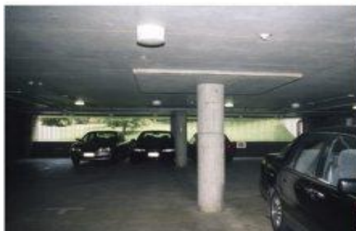
Fig. 9) Flat plate and Flat slab structural system
