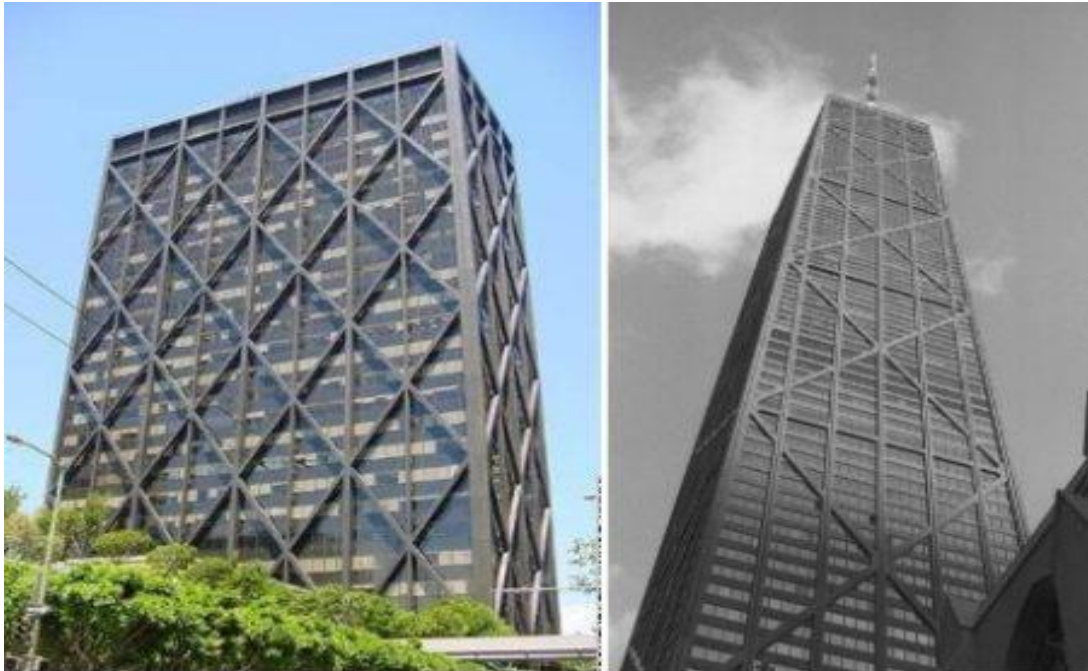
Fig.3) Braced Frame structural system
