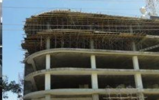
Fig. 9) Flat plate and Flat slab structural system
