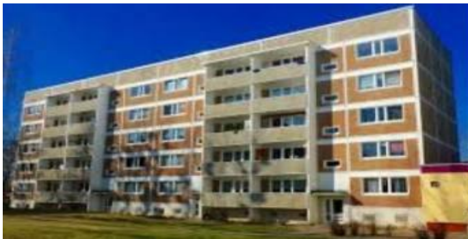
Fig.8) In Filled Frame structural system
