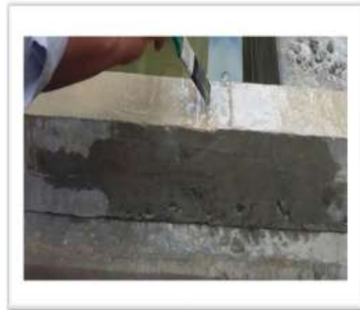
Fig. 6 Applying Resin over Surface of Beam
