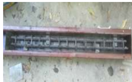
Fig. 2 Reinforcement in Steel Mould
