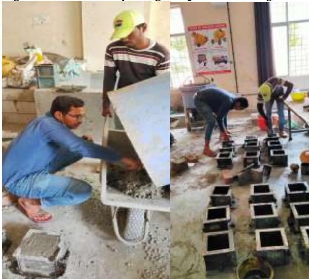
Fig: Concrete cube casting by using Polypropylene Fiber and Steel fiber in the moulds.
